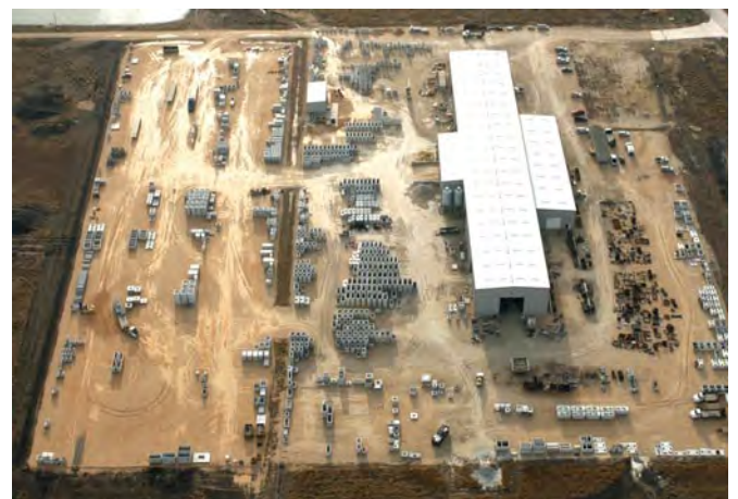
Figure 2: The new 46-acre Capital Precast facility in San Marcos, Texas, provides room for growth. The 50,000 s.f. production building features multiple bridge cranes and an ACT MobilMat batching system, allowing the use of SCC mix for products ranging from junction boxes and inlets to electrical manholes and septic tanks.
