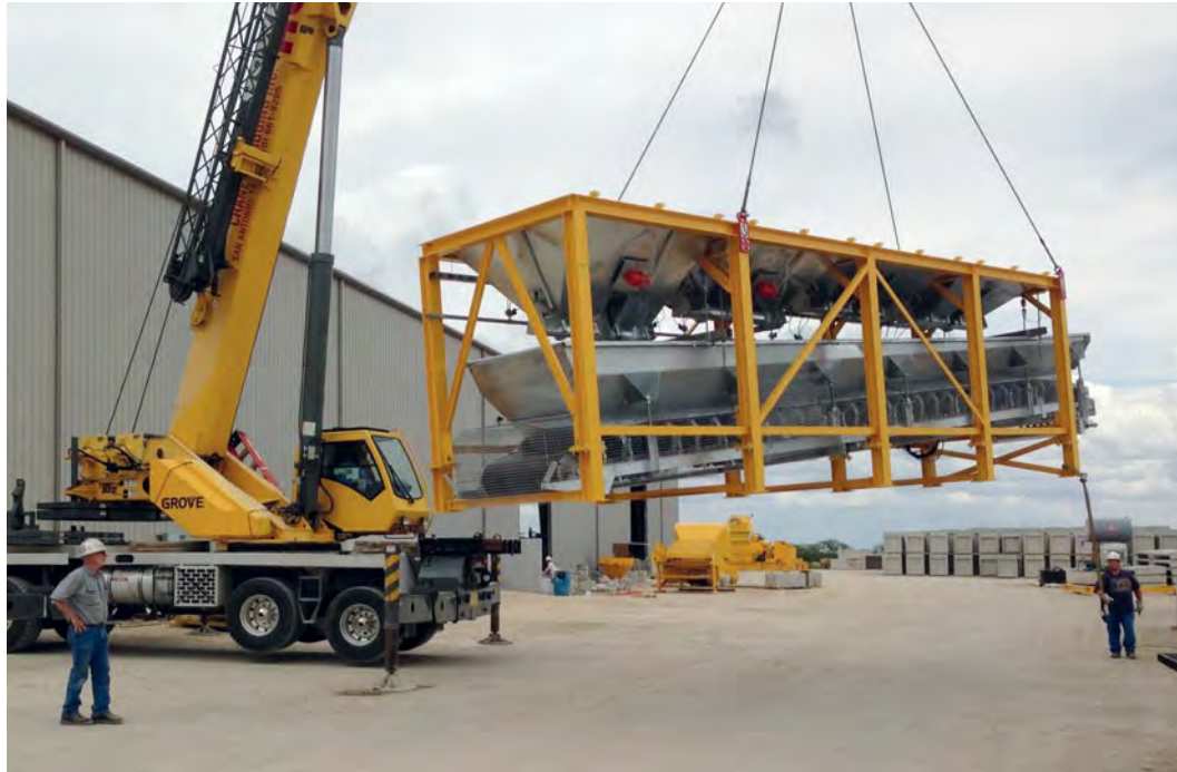
Figure 7: Four-compartment aggregate bin base section and weigh belt conveyor arrive as pre-tested modular unit for easy installation. Galvanized cones shown here provide extended life and lower operating costs. Ash's father Bill Wineinger (at left) helps direct the operation.
